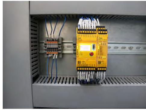
Picture 27 Hazard 3.3, Image 2, PILZ PNOZ m B0 safety controller with PNOZ S7 safety contact expansion
