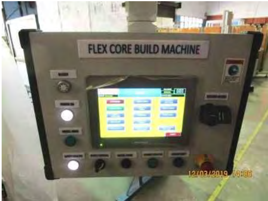
Picture 20 Hazards related to the control system
