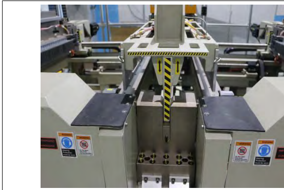
Picture 28 Hazard 3.4, Image 1, Light curtain installed at 342 mm
