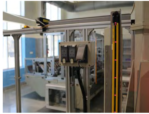
Picture 8 Hazard 1.5, Image 2, Safety magnetic door switch
